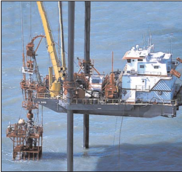
Figure 9: CT Operations from a Liftboat
