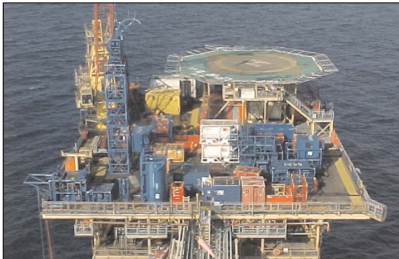
Figure 11: CT Operations on an Offshore Platform
