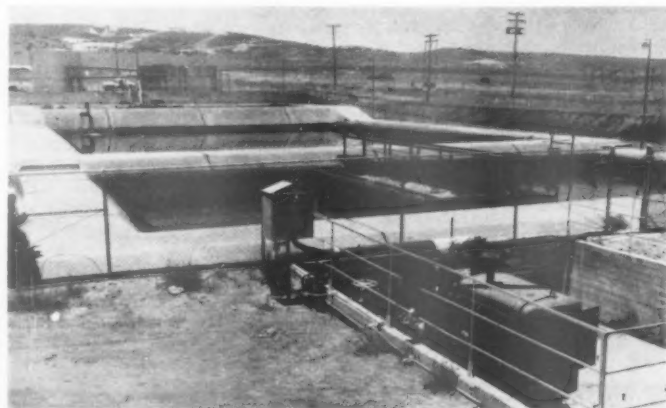
RICHFIELD OIL CORP. uses this central disposal pit for getting rid of its brine in South Cuyama field. Daily brine production is about 3,500 bbl. daily.
